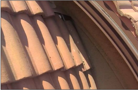
TILE ROOFS Concrete Tile Installation
