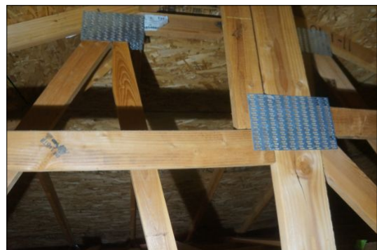
ATTIC Roof Structure- Trusses
