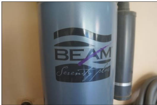
GENERAL INTERIOR General Condition
