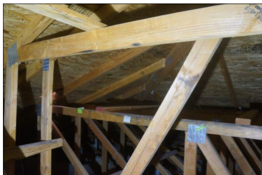
ATTIC Roof Structure- Trusses
