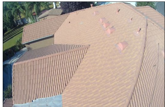
TILE ROOFS Concrete Tile
