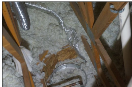
ATTIC Ventilation Condition
