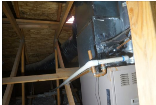
ATTIC Attic General Condition
