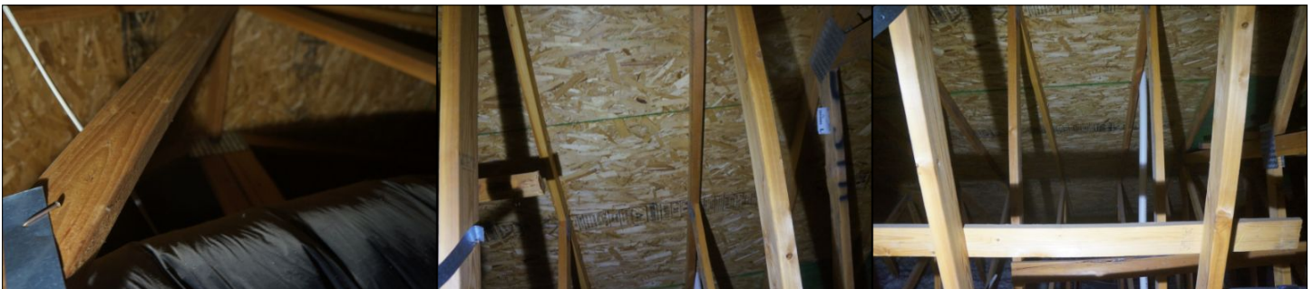
ATTIC Roof Structure- Trusses
