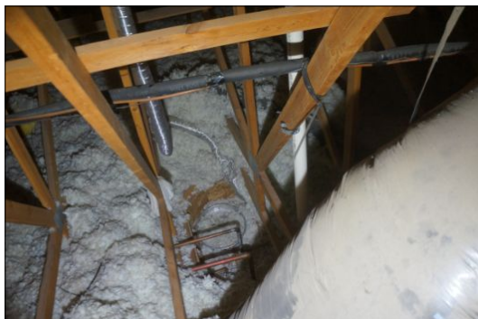
ATTIC Ventilation Condition
