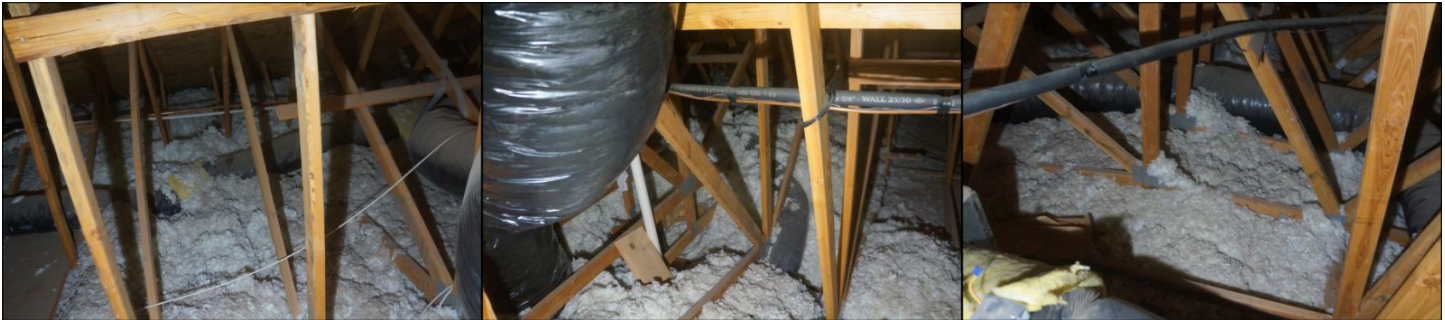
ATTIC Insulation Condition
