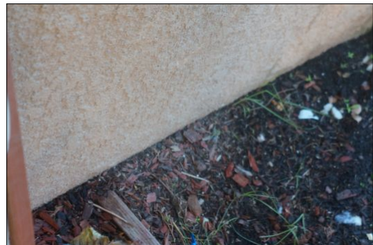
EXTERIOR WALLS Stucco/EIFS Instillation
