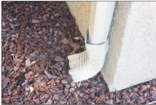
EXTERIOR ROOF STRUCTURE Roof Drainage System
