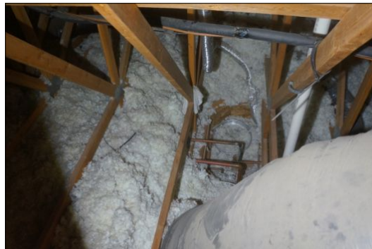
ATTIC Insulation Condition
