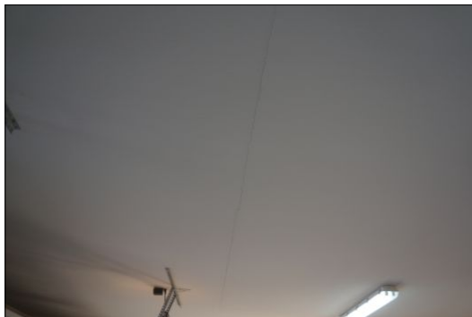
GARAGE Garage Ceiling
