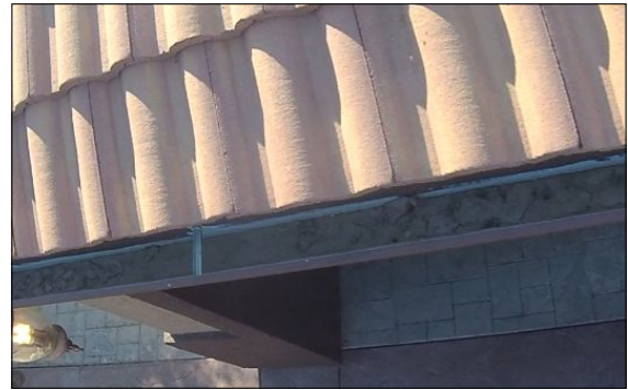
EXTERIOR ROOF STRUCTURE Roof Drainage System
