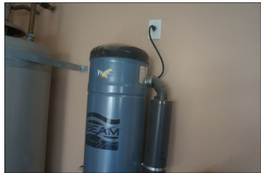
GENERAL INTERIOR General Condition
