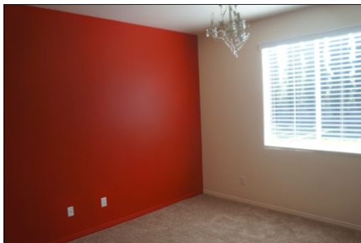
BEDROOM 4 General Condition
