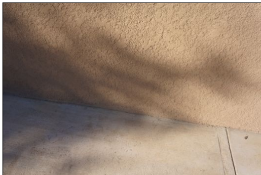
EXTERIOR WALLS Stucco/EIFS Instillation
