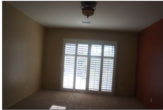
MASTER BEDROOM General Condition
