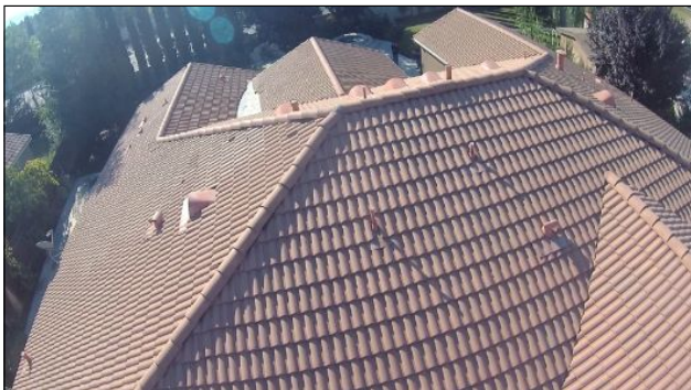
TILE ROOFS Concrete Tile
