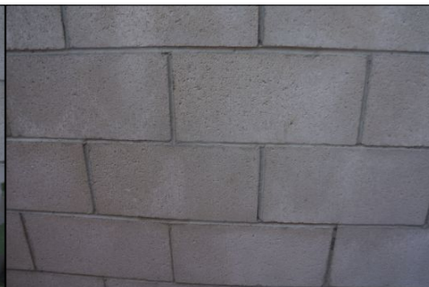
GROUNDS Masonry Walls
