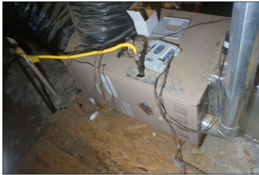
FURNACE General Condition
